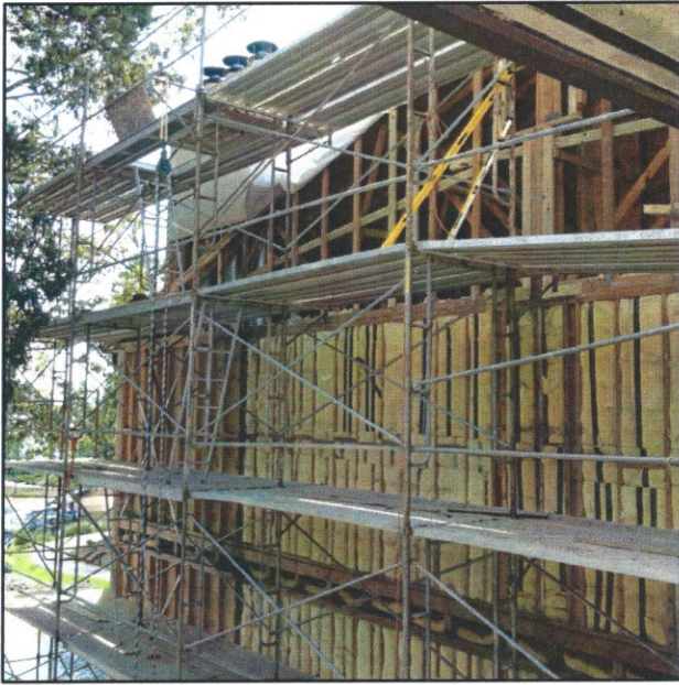
Views of existing framing and insulation with new plywood sheathing starting at the bottom.
