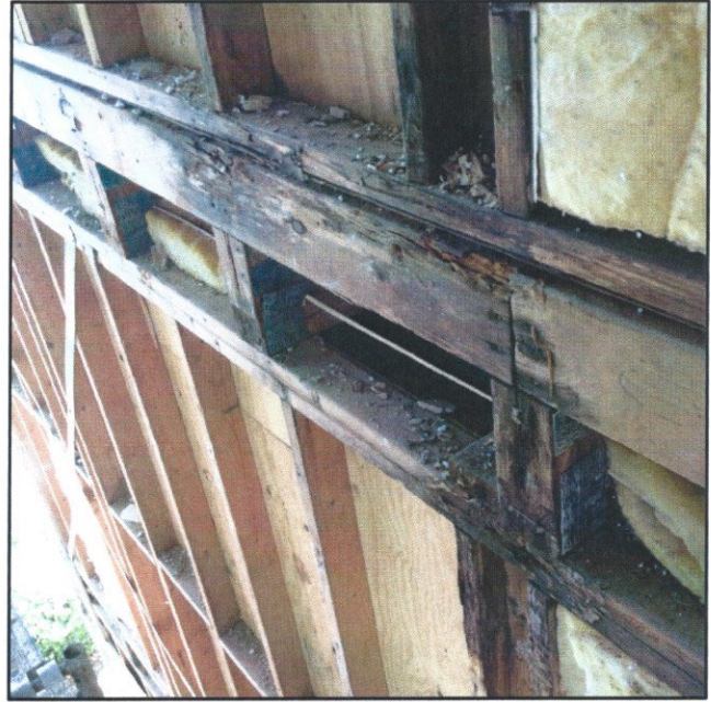
Views of damaged framing at floor to wall intersection and below the attic louver. This framing will be replaced.
