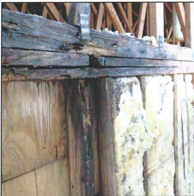
Views of damaged framing at floor to wall intersection and below the attic louver. This framing will be replaced.
