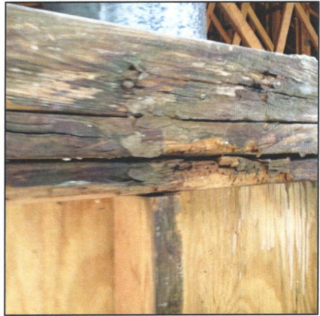
Views of damaged framing at floor to wall intersection and below the attic louver. This framing will be replaced.
