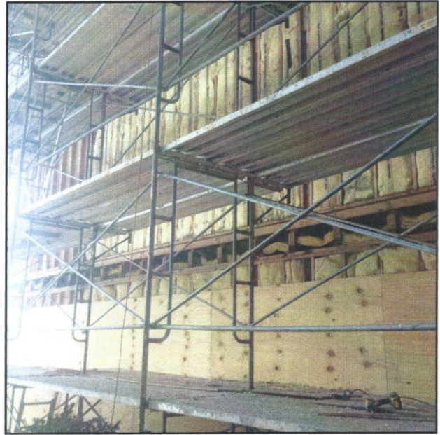
Views of existing framing and insulation with new plywood sheathing starting at the bottom.
