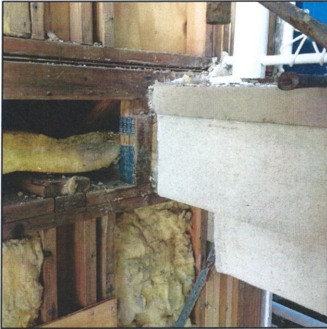
Views of damaged framing at floor to wall intersection and below the attic louver. This framing will be replaced.
