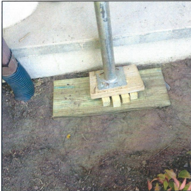
Views of shoring posts installation in progress.
