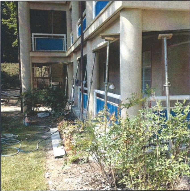
Views of shoring systems secured in place. Temporary dust barriers are in place.
