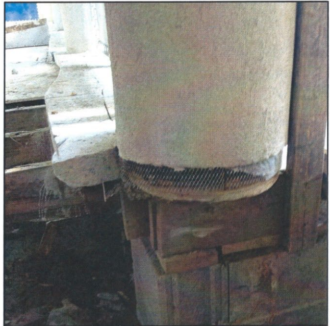
Views of temporary access walkway to Unit 101. Views of deteriorated wood condition under columns and at wall.
