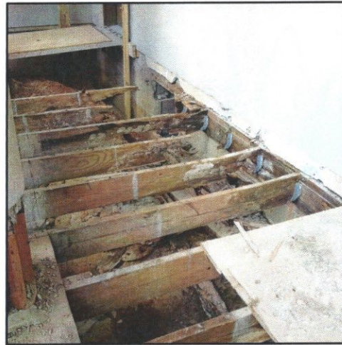
Views of work in progress at column bases and removal of floor wood framing.
