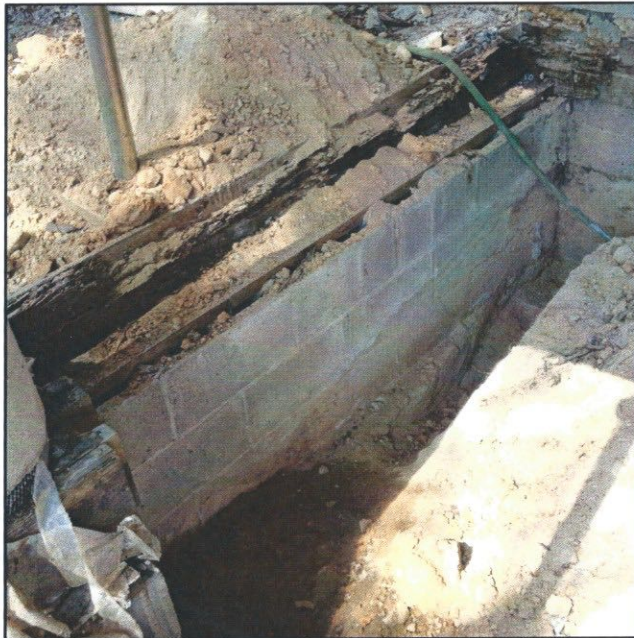
Views of temporary access walkway to Unit 101. Views of deteriorated wood condition under columns and at wall.
