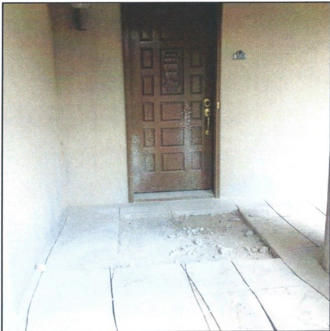
Views of rotted wood framing and concrete removal in progress.
