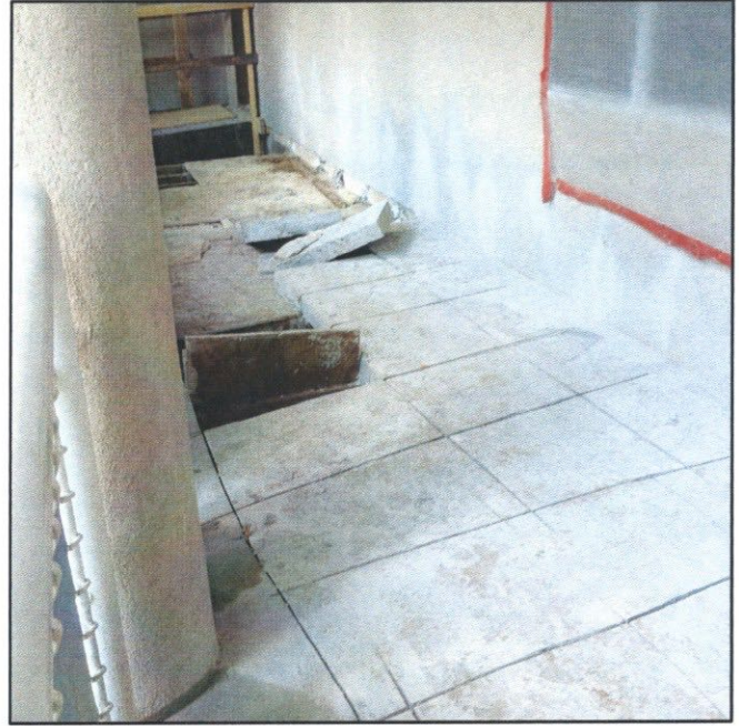
Views of rotted wood framing and concrete removal in progress.
