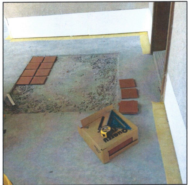
Views of floor cut out prepared to receive new terra cotta tile.
