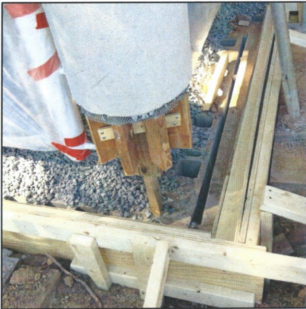
Views of installation of the washed stone sub base and edge form work.
