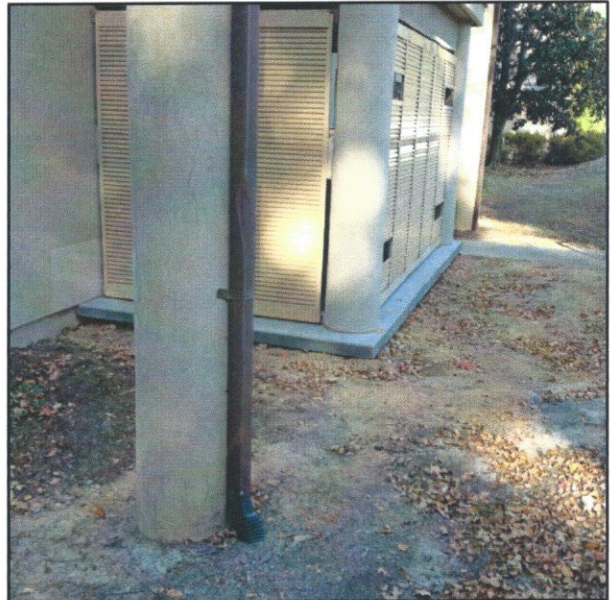
Views of new mechanical ventilation system at crawl space areas and the replacement of metal screen panels at stairways.
