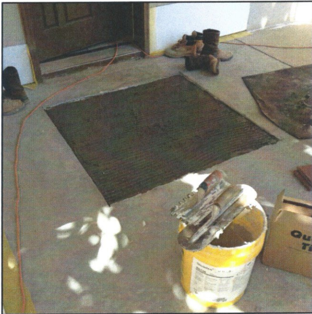
Views of terra cotta tile installation at the entrance doors of Units 101, 102 and 103. View at corridor showing work in progress to finish columns and new work at existing walls.
