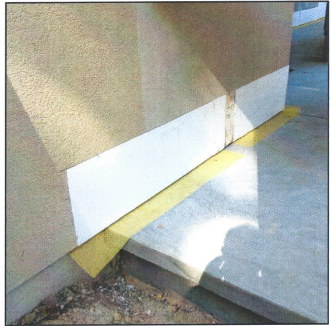
Views of new EIFS wall system being installed at floor.
