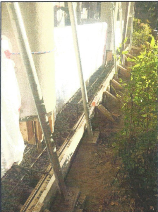
Views of reinforcing bars, washed stone and edge forms ready for pouring of concrete.
