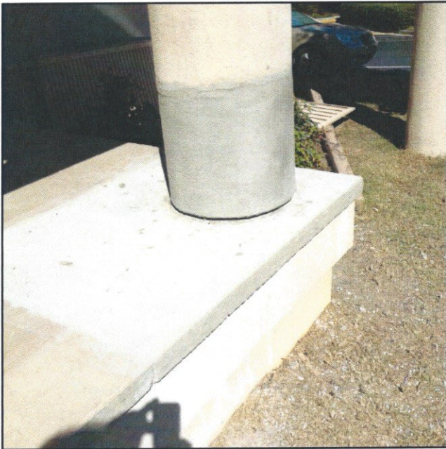
View of new stucco applied to corner columns.
