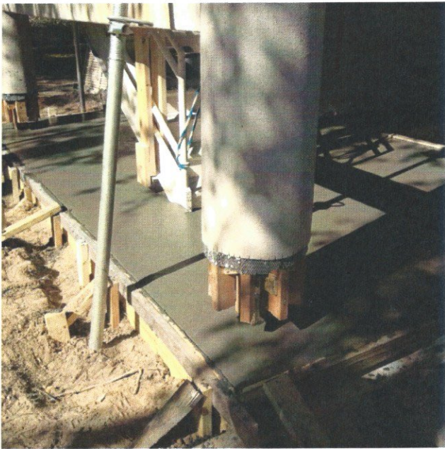
Views of new concrete pour at corner columns.
