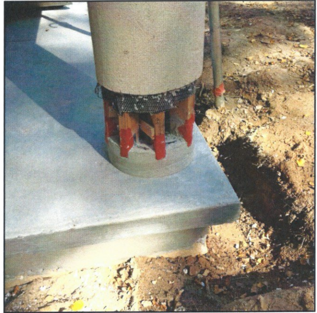
Views of new concrete curb at corner columns.
