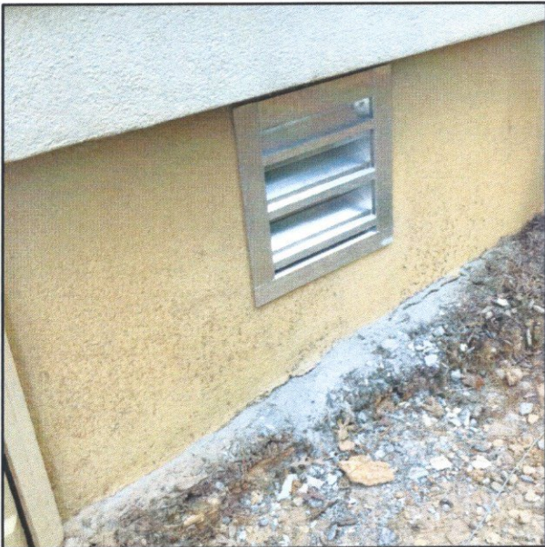
Views of new mechanical ventilation system at crawl space areas and the replacement of metal screen panels at stairways.
