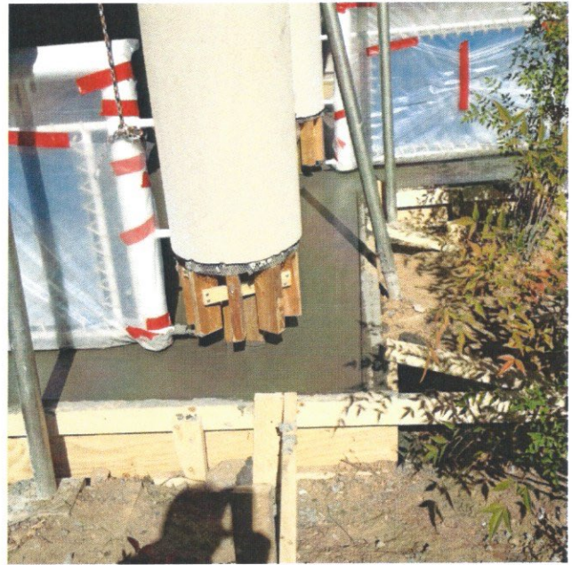
Views of new concrete pour at corner columns.
