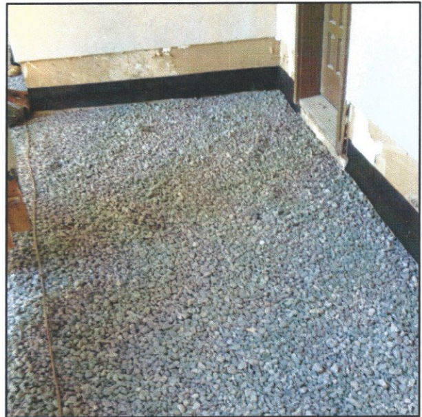
Views of installation of the washed stone sub base and edge form work.
