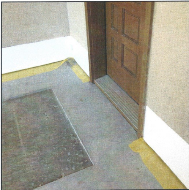
Views of floor cut out prepared to receive new terra cotta tile.
