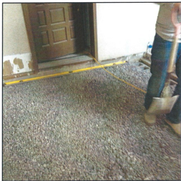
Views of installation of the washed stone sub base to support new concrete floor.
