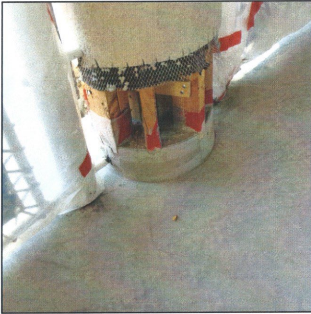
Views of new concrete curb at corner columns.
