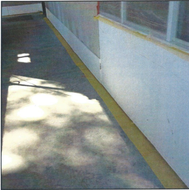
Views of new EIFS wall system being installed at floor.
